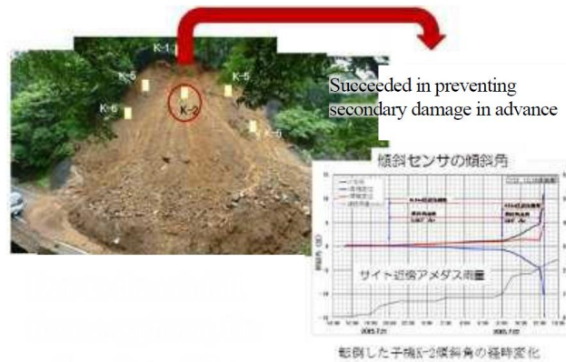
Figure 7.3.9 Equipment Installation Locations on the Cut Slope of the Damaged Road
