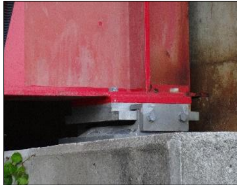
Bridge Pier and Bearing Part
