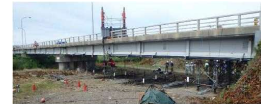
Full View of Load Testing
