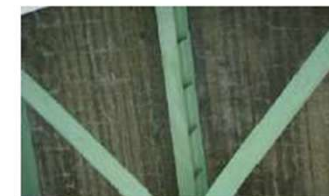
(a) Cracks in slabs
