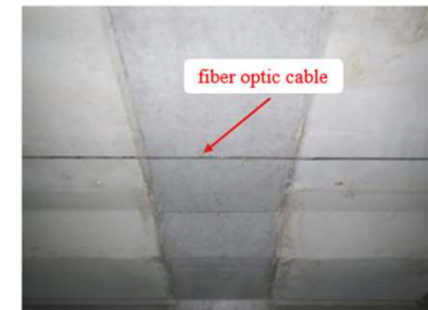
Underside of floor slab
