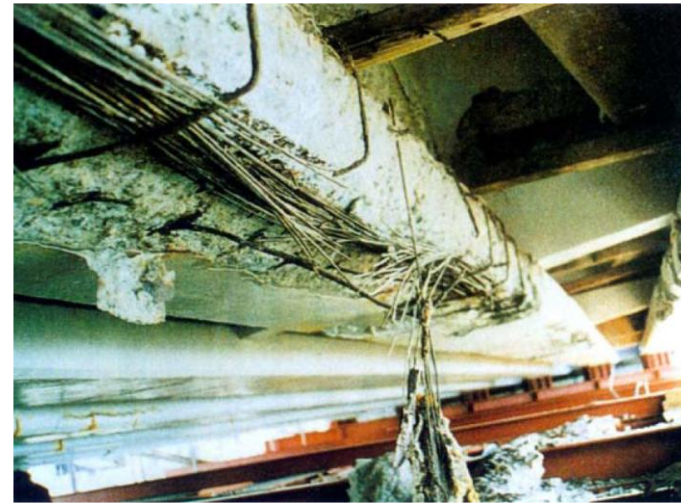
Deteriorated beam
