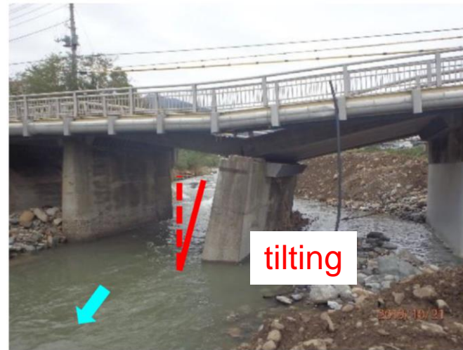
2019(terrible heavy rain) Inclination of piers
