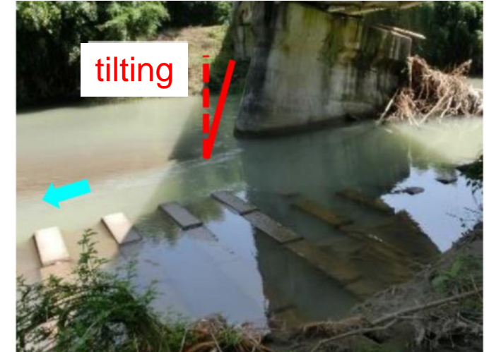
2019(terrible heavy rain) Inclination of piers
