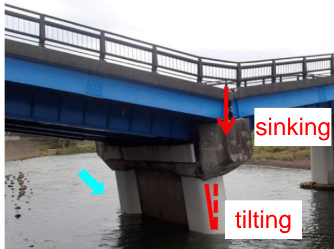
2021(terrible heavy rain) Subsidence of piers
