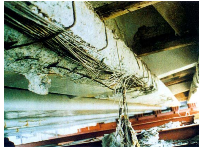
Deteriorated beam
