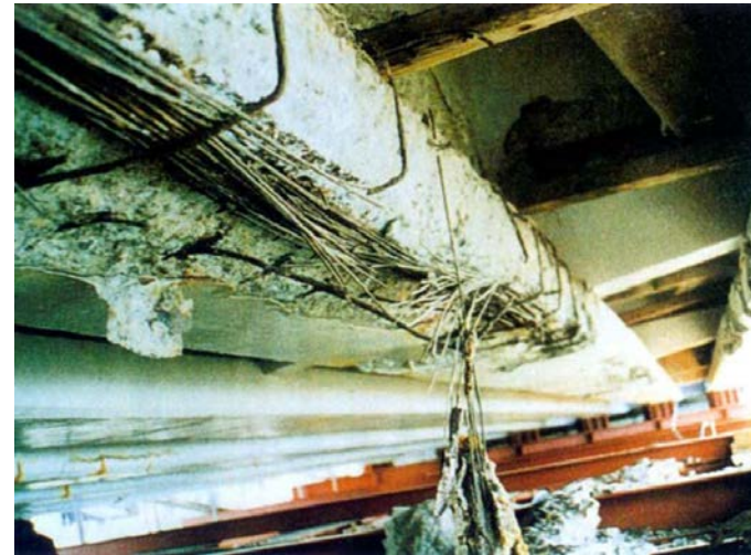
Deteriorated beam
