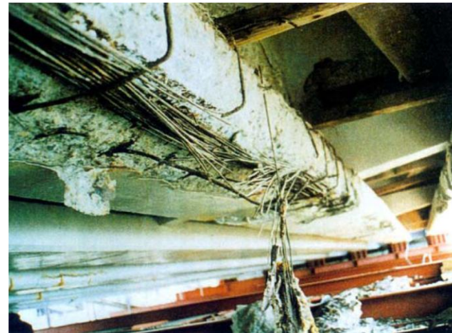
Deteriorated beam
